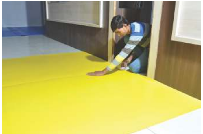
Temporary Floor Protection
